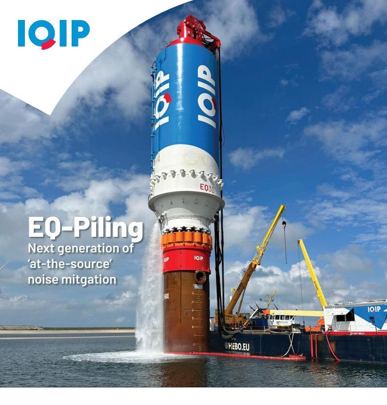
Reducing noise thanks to prolonged, gradual energy transfer. EQ-Piling leverages decades of experience with conventional impact hammers as well as nearfield and at-the-source noise reduction. IQIP's newly-developed approach allows you to meet even the most stringent environmental regulations and ensure marine life safety during installation without additional noise mitigation measures.
